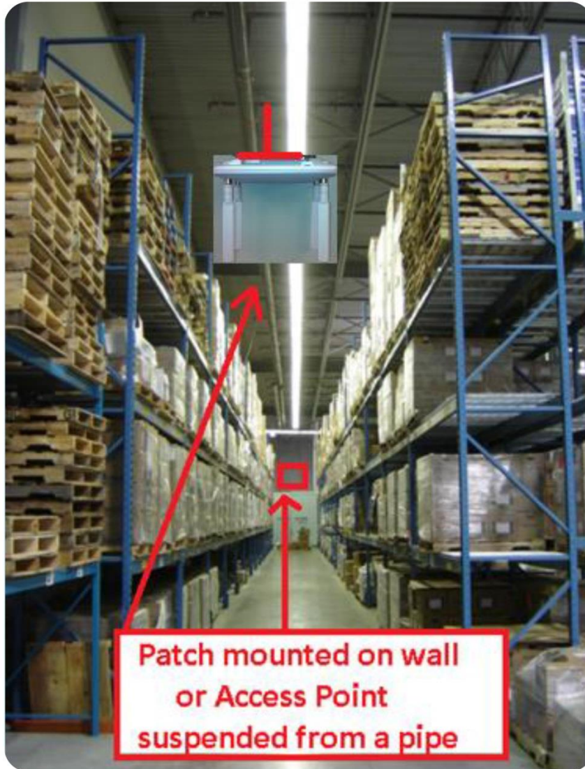
Figure 24. Access point placement in a warehouse environment (an external dipole “E” or internal antenna “I” could be used)
